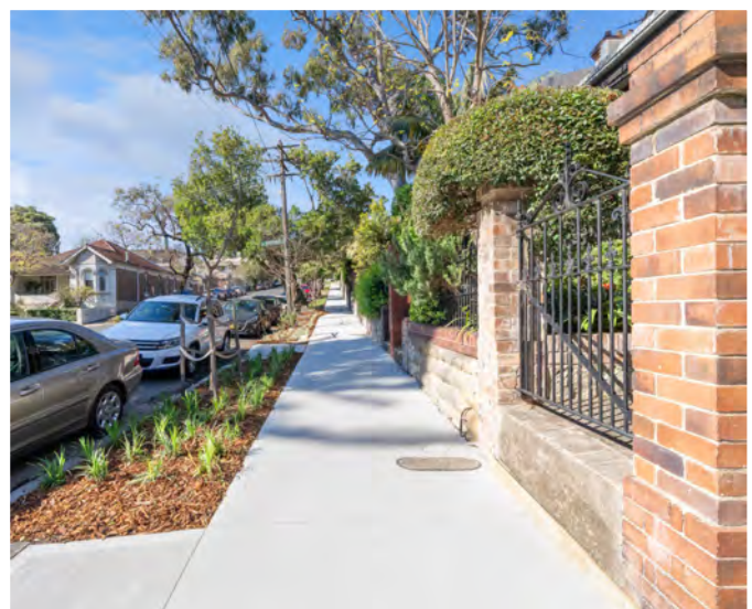
Images: Eglinton Road, Glebe Footpath Renewal Works 2021
